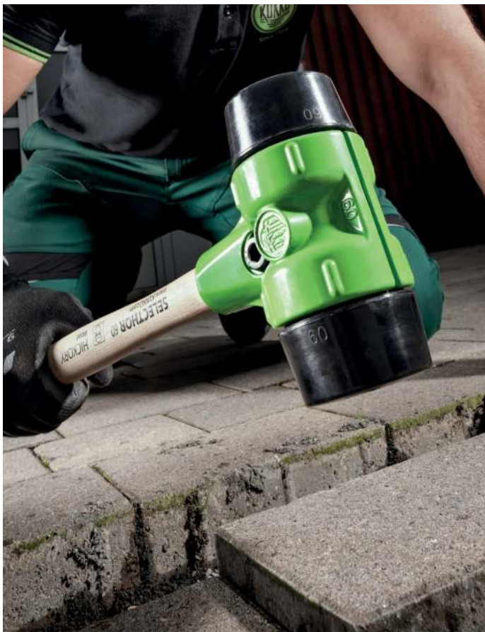
Use of a Selecthor soft-face hammer when laying paving stones
